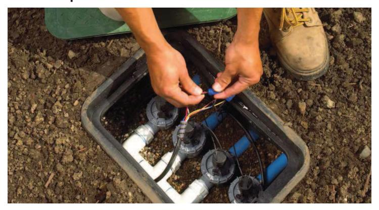
The Irritrol® 2400 Series globe and 2600 Series angle valves are popular with users because of the convenience of their threaded bonnets, the reliability of their double-beaded diaphragm and the durability of their heavy-duty, corrosion- and UV-resistant PVC construction. Fast and easy to install and service, these 1-inch residential plastic valves offer an encapsulated solenoid, internal/external bleed, an optional flow control feature, and are available in multiple configurations.
